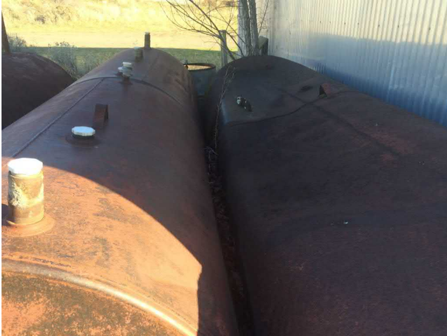
13. Waste oil tanks located beside hanger on west side of taxiway.
