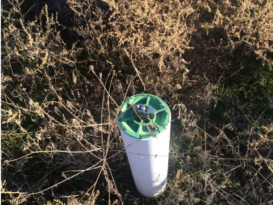
35. Septic system discharge valve.
