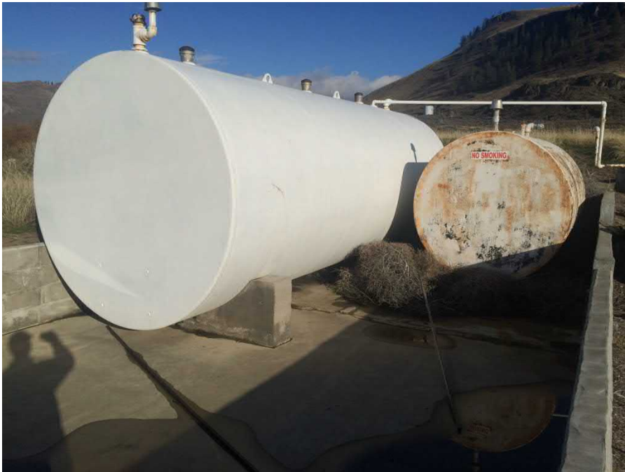
24. Above ground fuel storage tank & old UST on right (not presently used).
